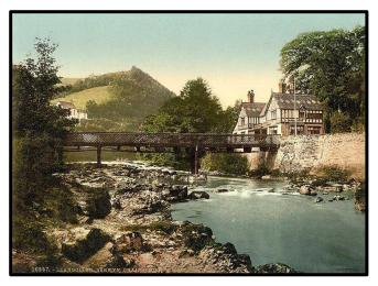
underneath the deck. The new design was a great improvement, being of higher strength and unaffected by floods because there was now no necessity for piers to stand on the river bed under the bridge in the middle of the river.
